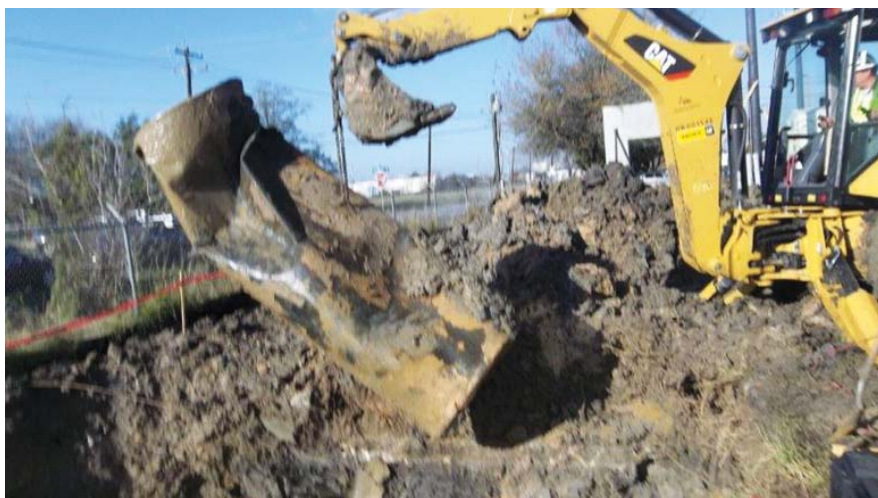
Removal of USTs in progress Removal of USTs in progress – Photographs by Kevin Casler
